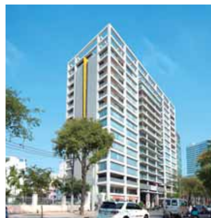
The Landmark, Ho Chi Minh City, Vietnam (office and residential) Established: 1994
