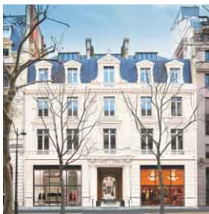
21 avenue Kléber Paris, France (office and retail) Acquired: 2013
