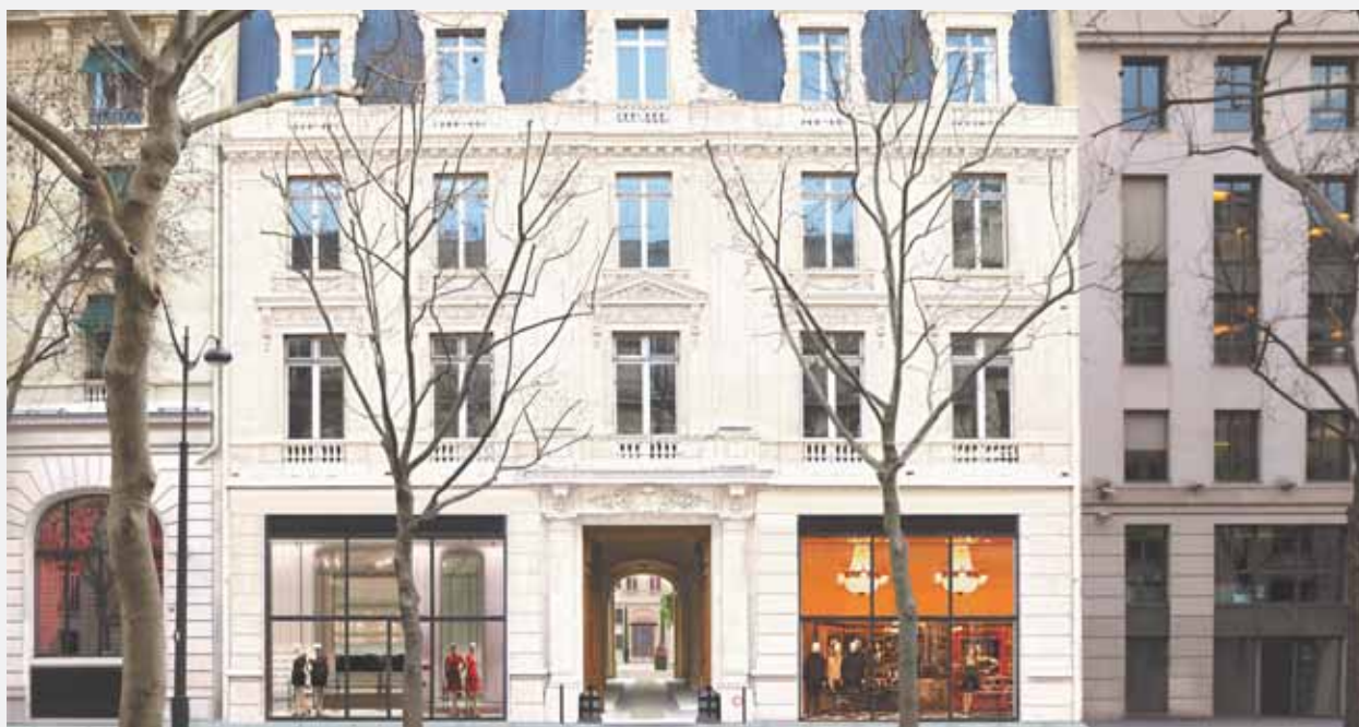
A spectacular renovation of 21 avenue Kléber, Paris was completed and leases were signed with major office and retail tenants.
