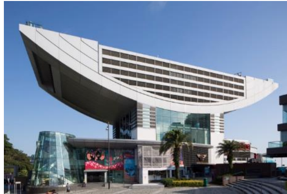
THE PEAK TOWER, HONG KONG
