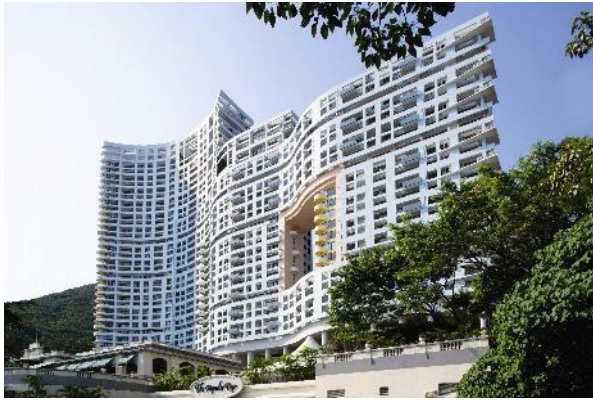
THE REPULSE BAY COMPLEX, HONG KONG
